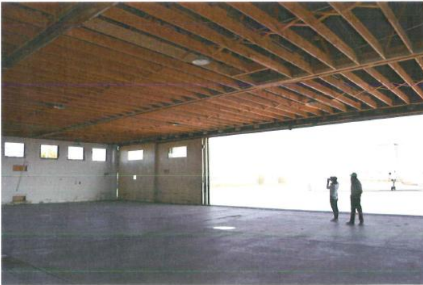
Airport Hangar #2, May 19, 2014
