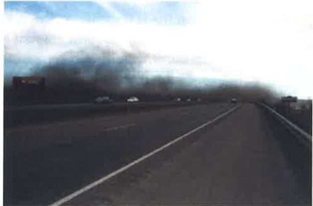
Coal dust from the coal pile at Corette power plant blows across the interstate outside Billings.
