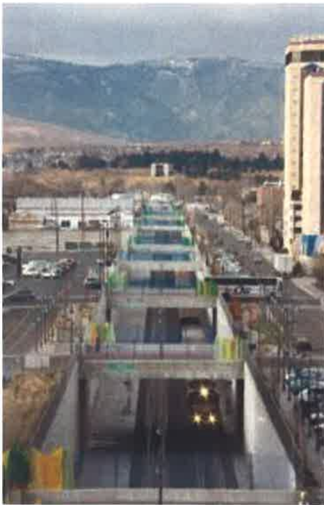
Reno, NV lowered the rail line that runs through the city in order to reduce traffic delays.
